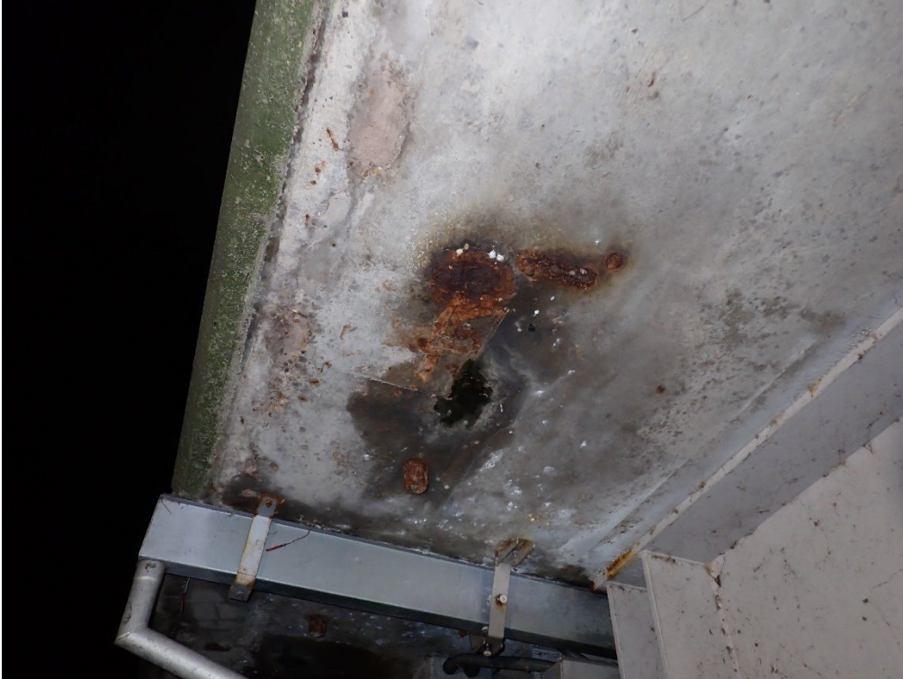
Plate 109. Minor spall to the North edge beam adjacent the Centre Joint
