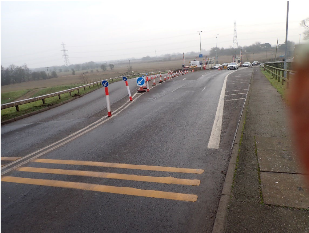
Plate 30. View East of structure
