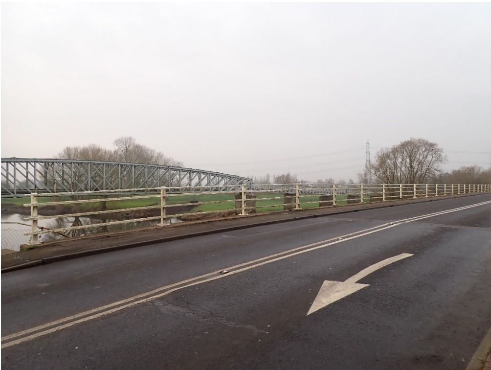
Plate 28. South Parapet, East
