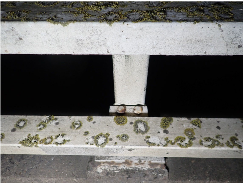
Plate 168. Typical lichen growth on the Parapets
