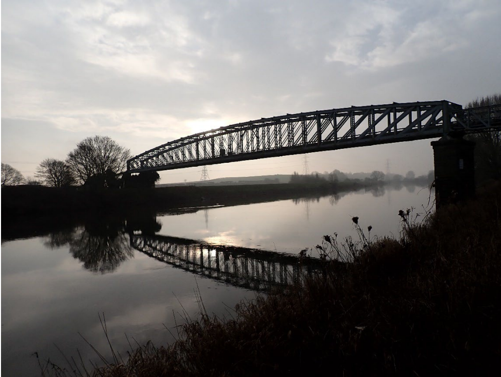
Plate 31. View upstream of structure
