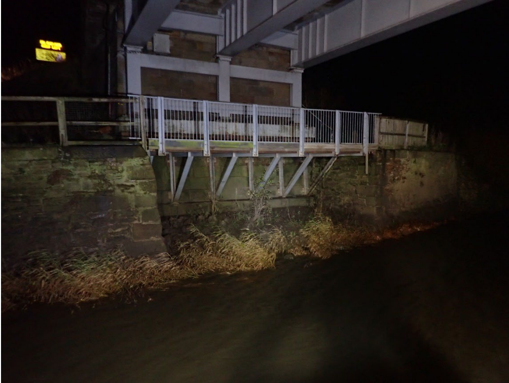
Plate 33. East Riverbank and Retaining Wall
