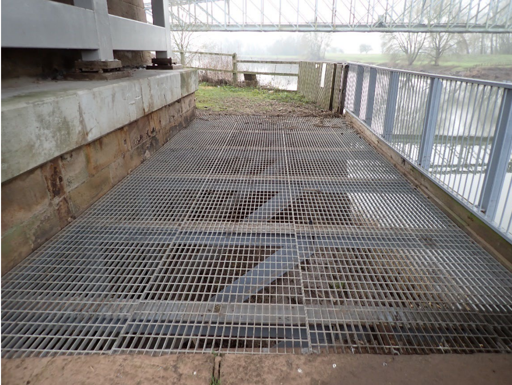
Plate 35. East Abutment walkway
