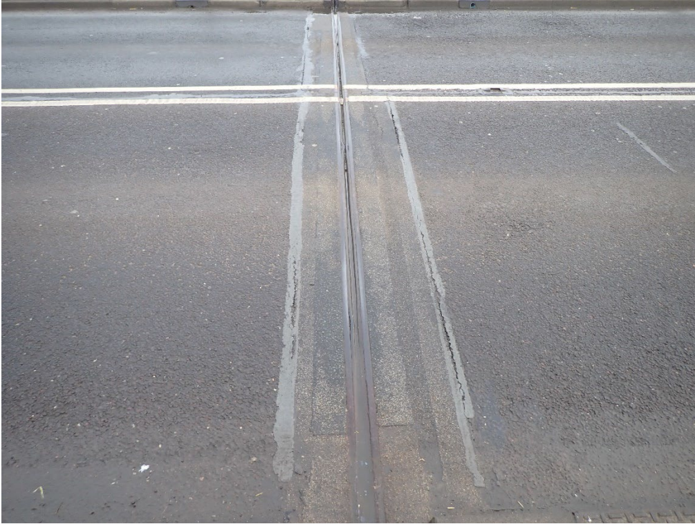
Plate 23. East Pier Expansion Joint
