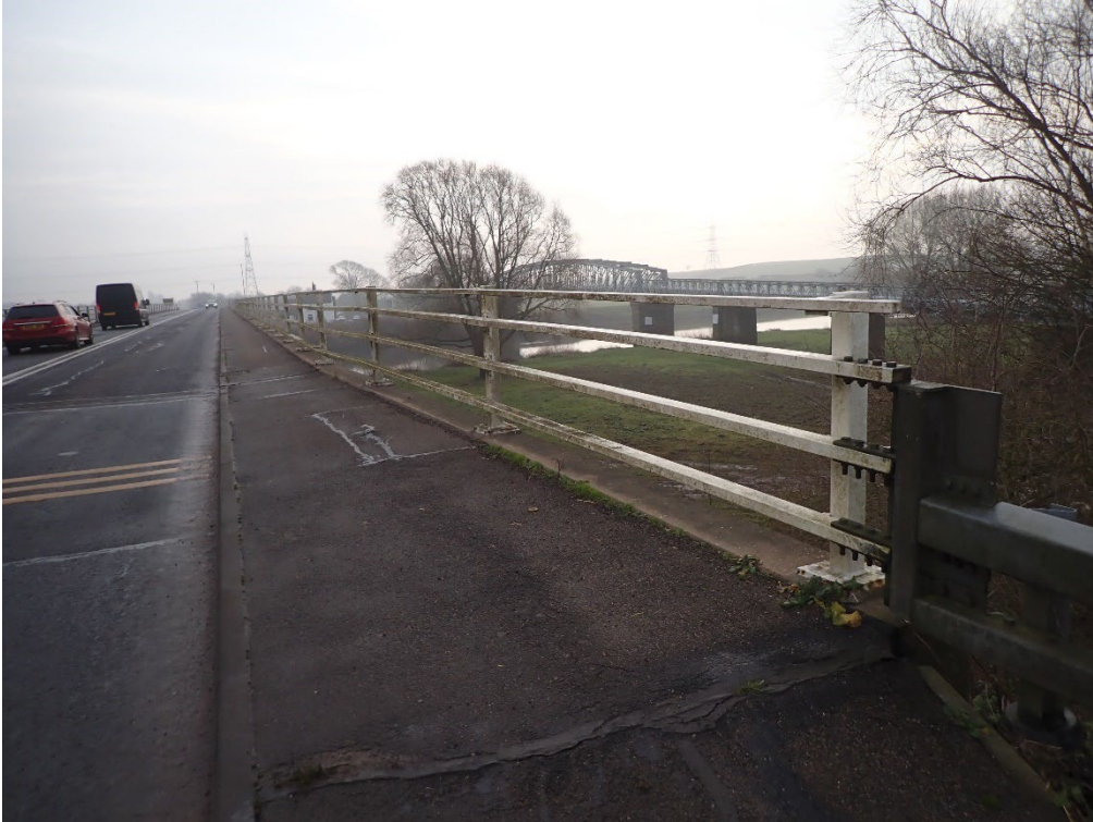
Plate 27. South Parapet, West
