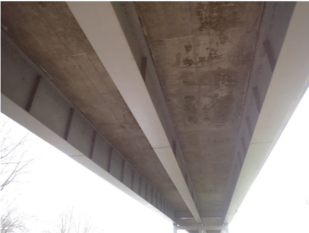
Plate 14. Outer West Span Soffit
