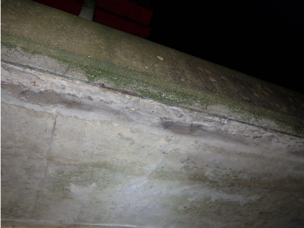
Plate 123. Long narrow repair, inner West Span, South Cantilever Soffit
