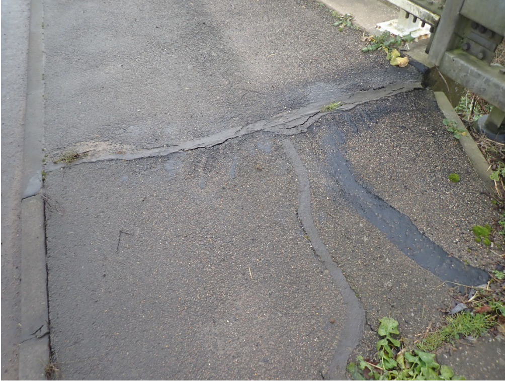
Plate 157. Surface and cracking repairs at the West end of the South Footpath on the approach
