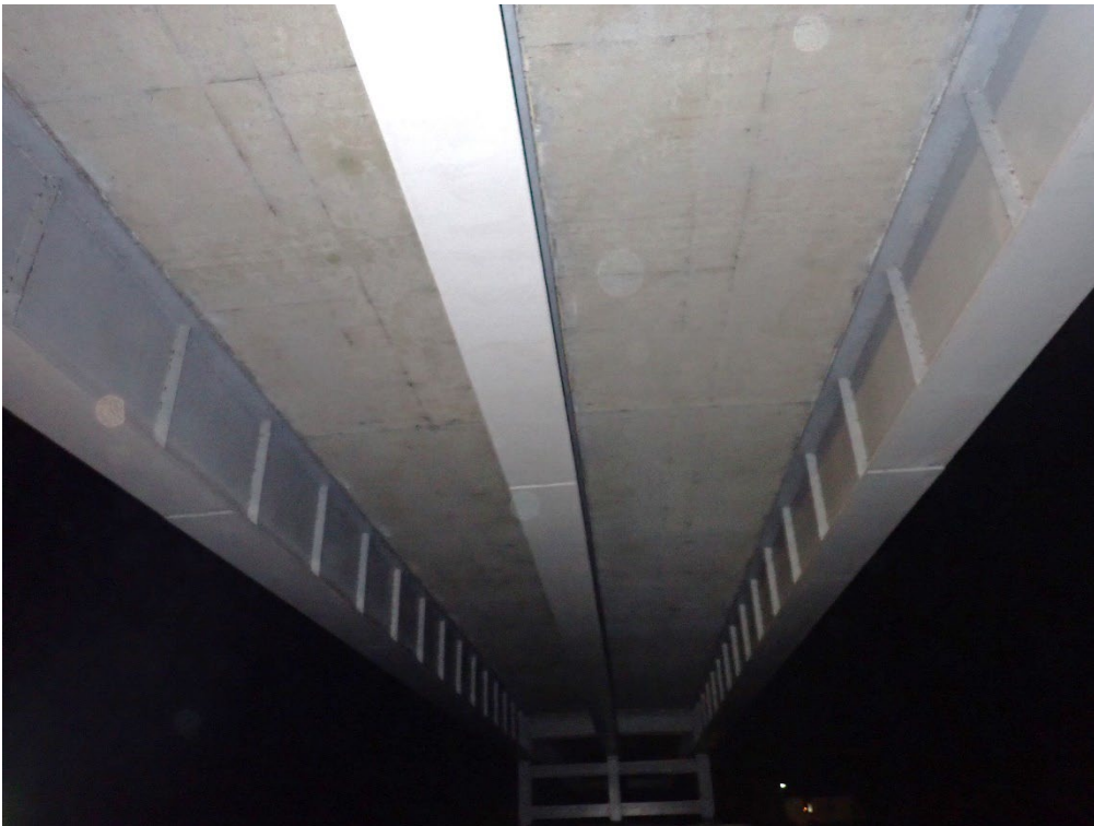
Plate 16. Inner East Span Soffit
