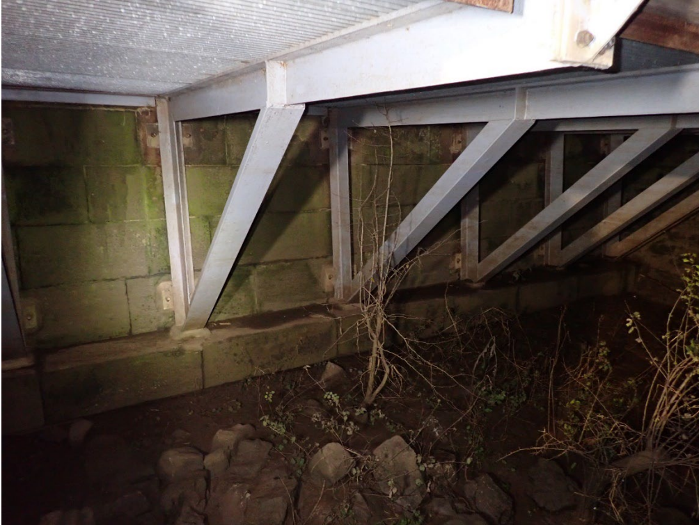
Plate 177. Typical Condition of Walkway Frame
