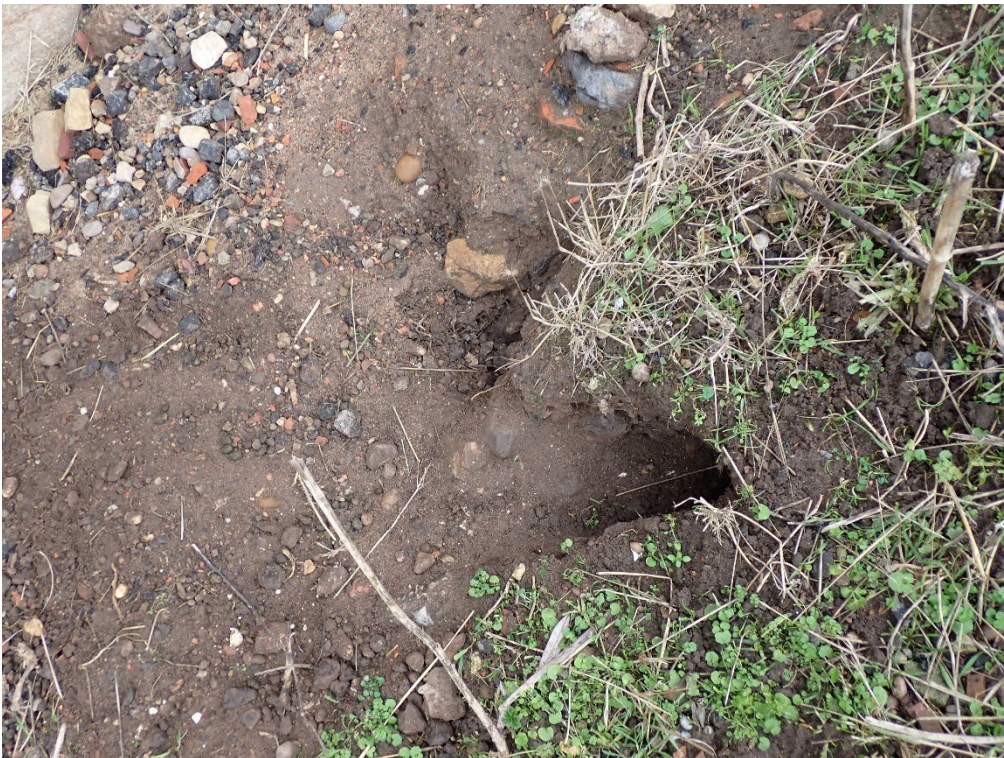
Plate 172. Animal burrows on the bank adjacent to the North-East Wing Wall
