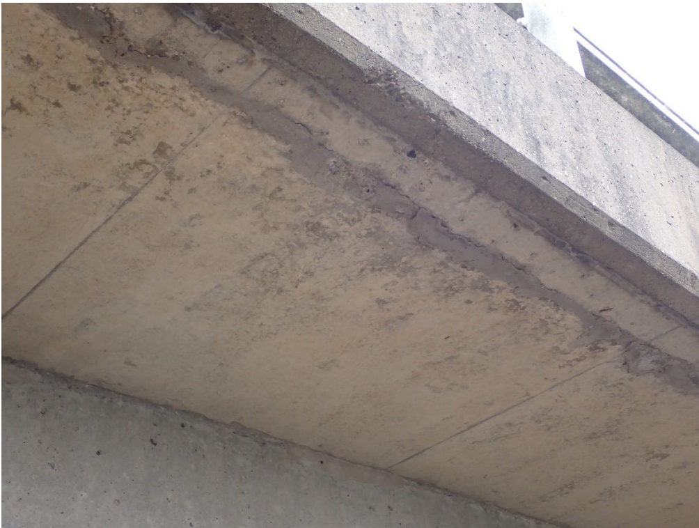
Plate 122. Typical view of narrow repair in Cantilever Soffit, South-East corner
