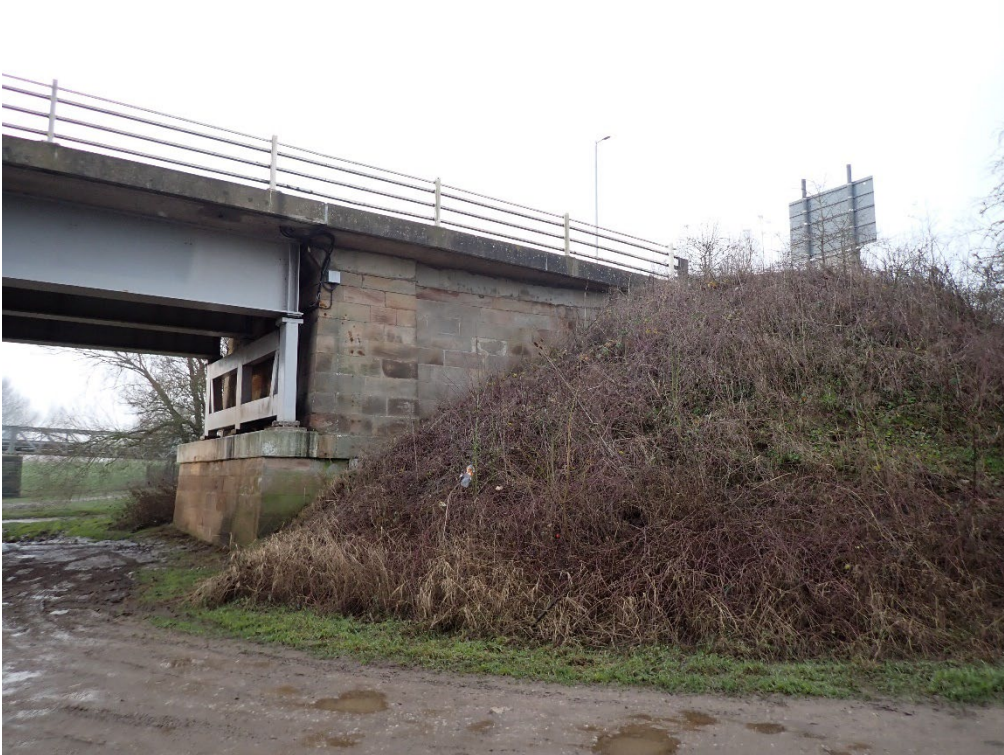
Plate 5. North-West Wing Wall
