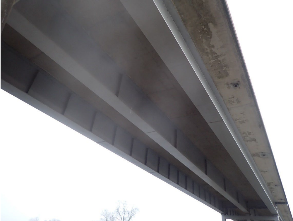
Plate 15. Inner West Span Soffit
