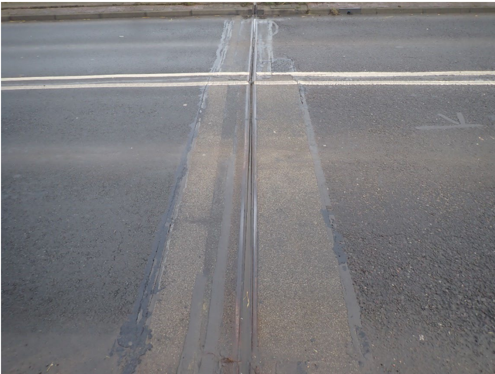
Plate 20. West Expansion Joint
