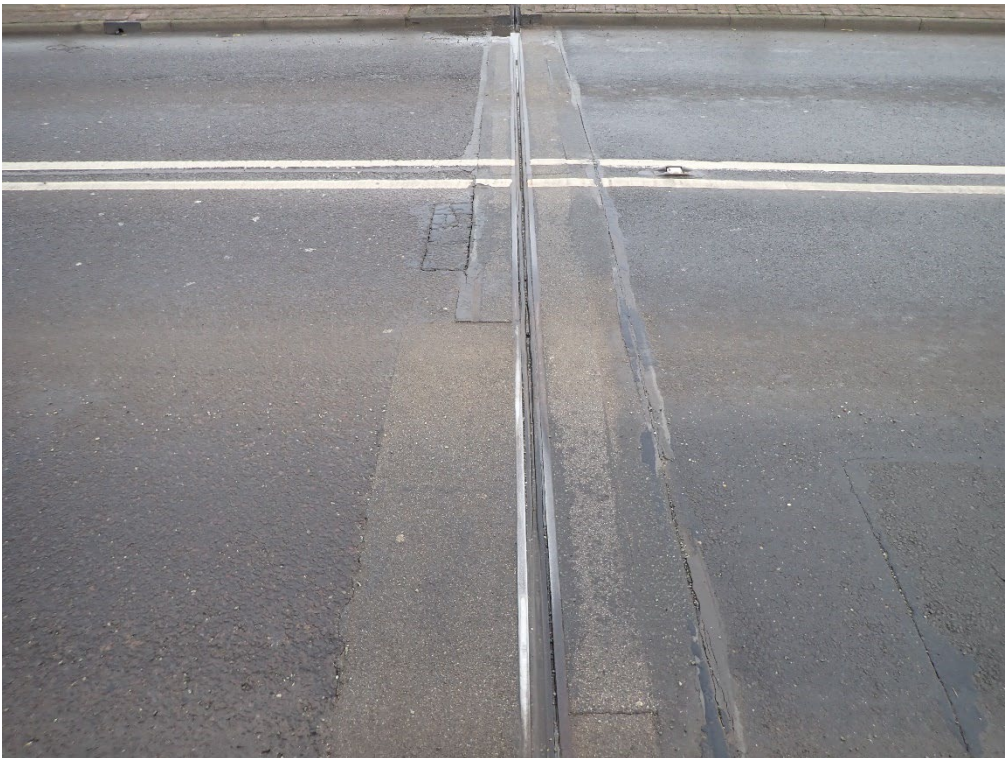
Plate 24. East Abutment Expansion Joint
