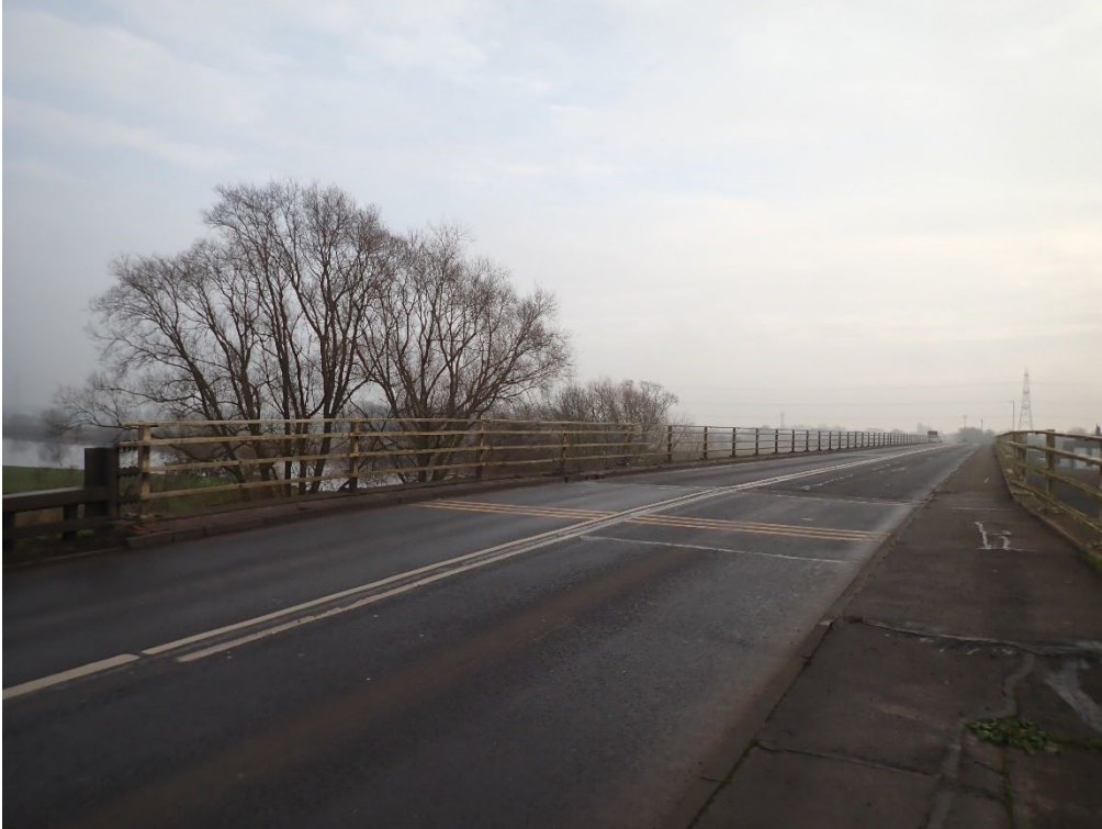
Plate 25. North Parapet, West
