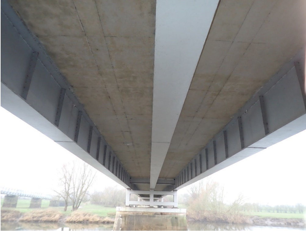
Plate 17. Outer East Span Soffit
