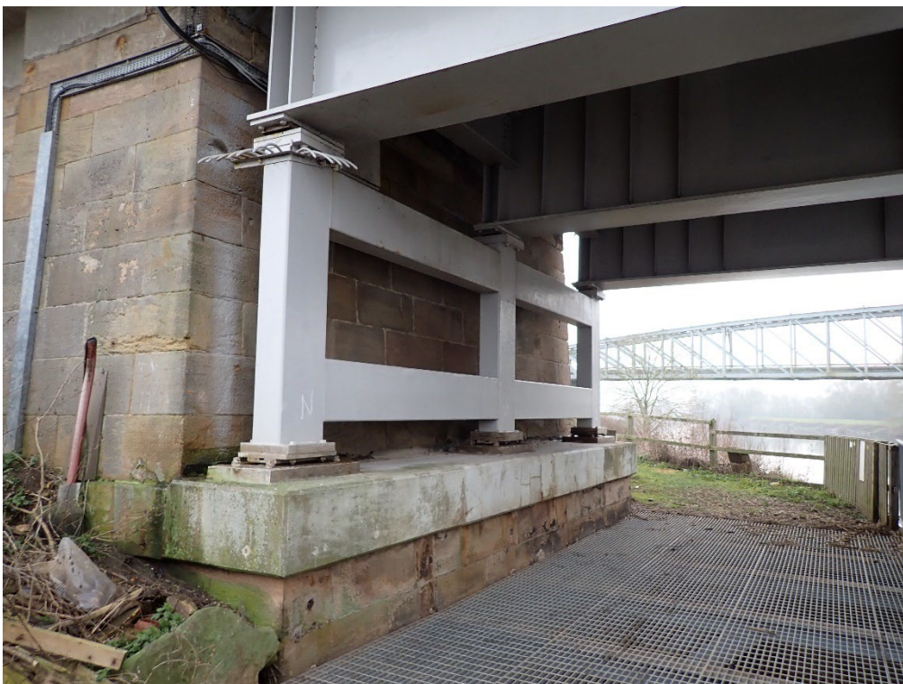
Plate 40. Repair to front face of East Abutment concrete cap
