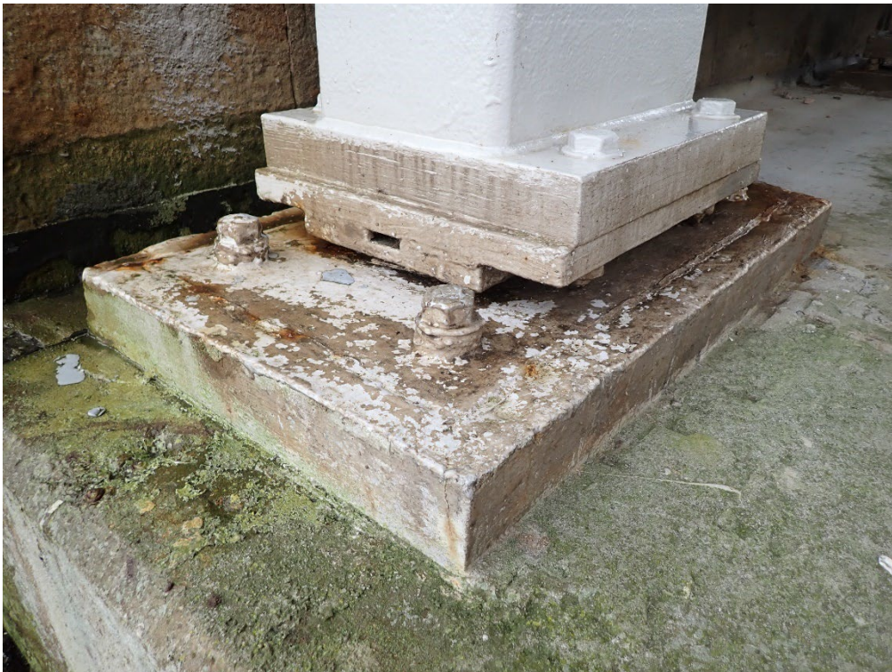
Plate 12. Typical lower Bearing, East Abutment
