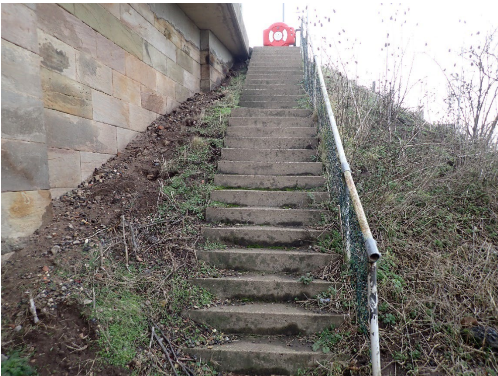
Plate 34. Access Stairs to the South-East of the structure
