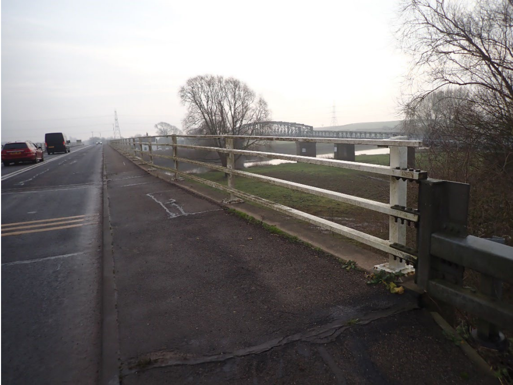
Plate 161. Repair to Crack in the South Footpath
