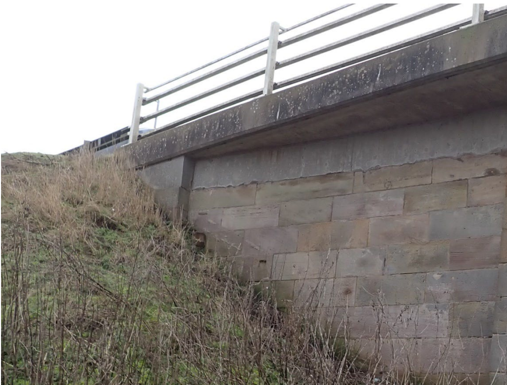
Plate 64. Evidence of Old Cable Tray, North-East Wing Wall
