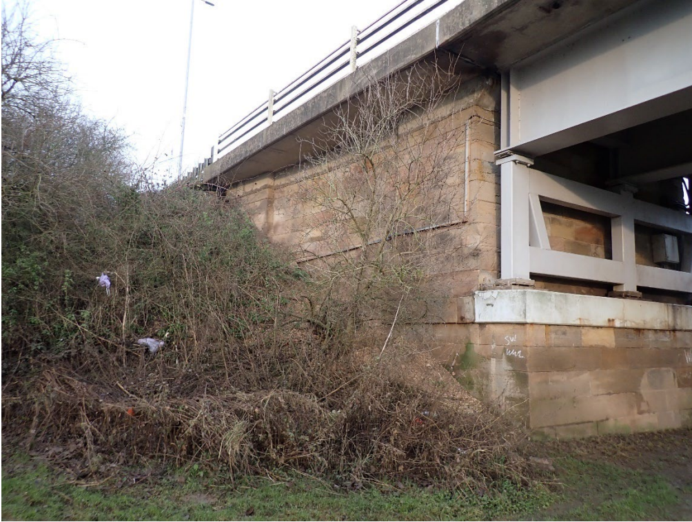
Plate 7. South-West Wing Wall
