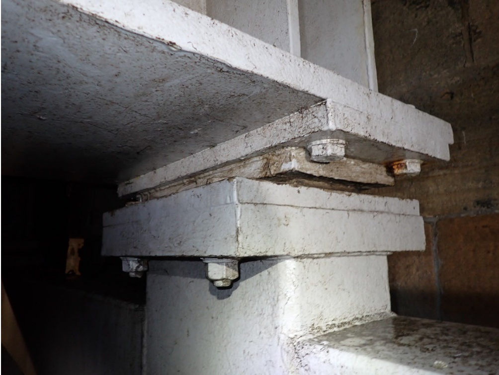
Plate 13. Typical Upper Bearing, East Abutment
