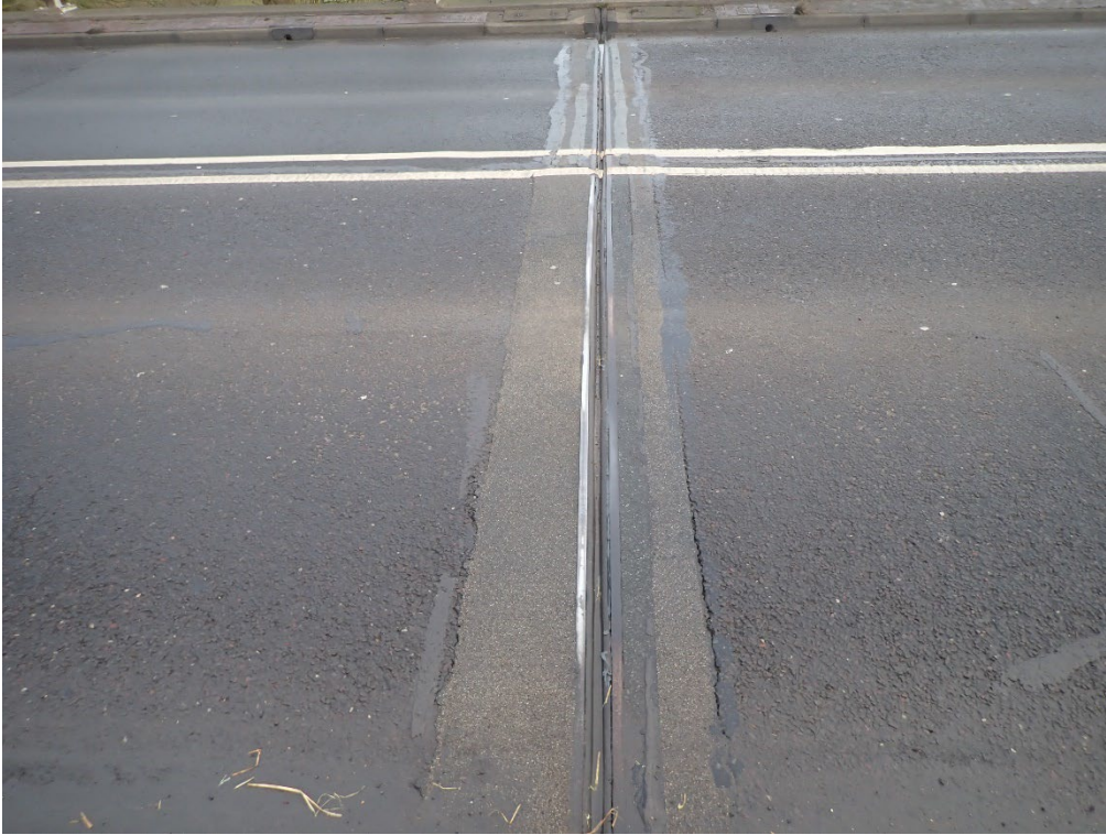
Plate 21. West Pier Expansion Joint
