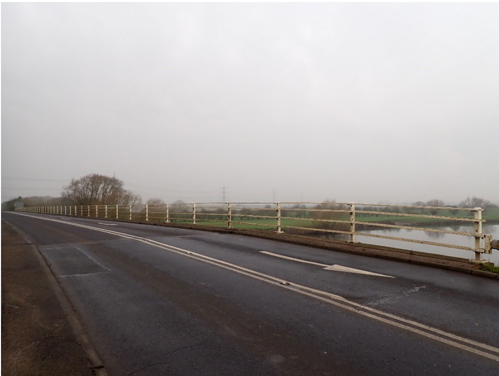
Plate 26. North Parapet, East
