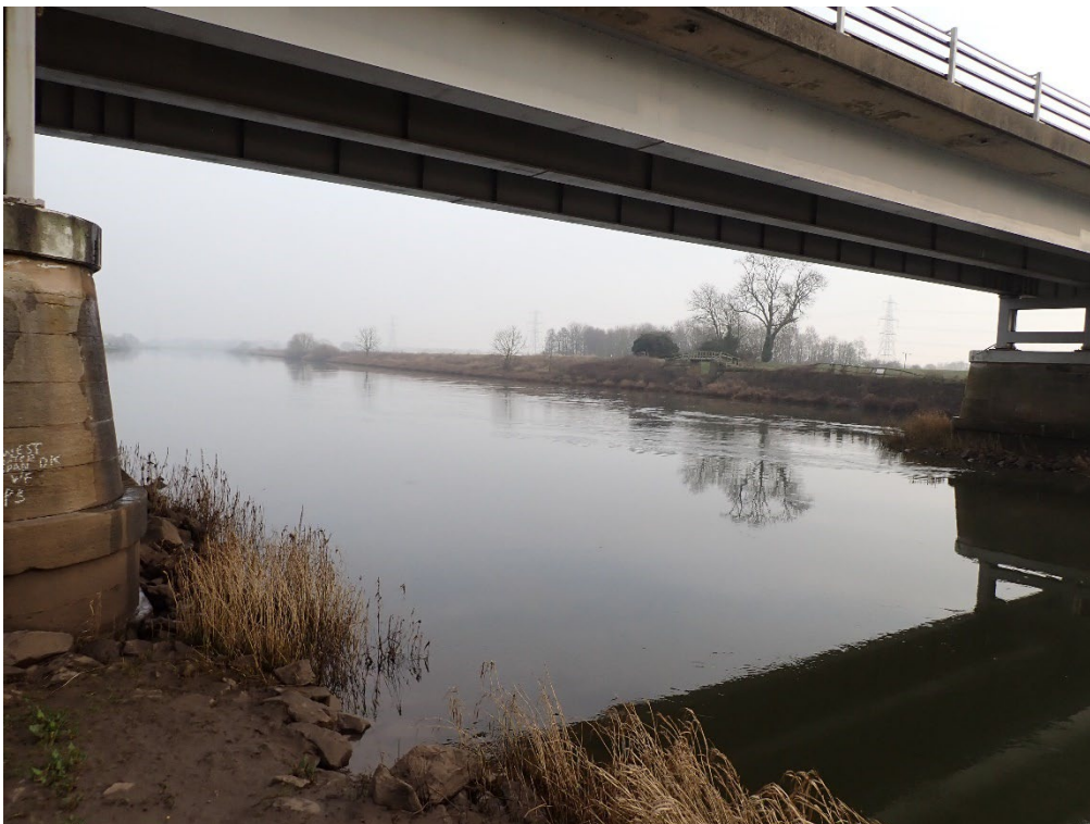
Plate 32. View downstream of structure
