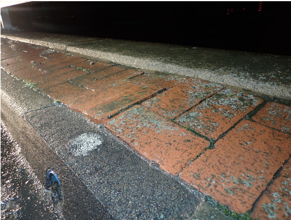
Plate 162. Movement of bricks at drainage locations in North Verge
